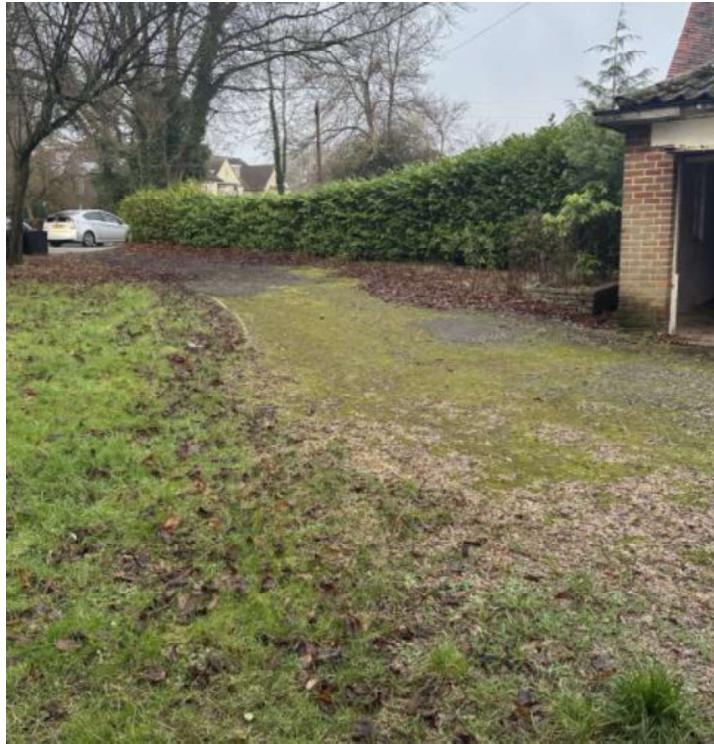
Figures 6: Showing existing hardsurfacing, access arrangements and garage
